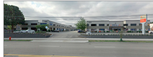
BLDG. 300 & 400 View from 80 Avenue
