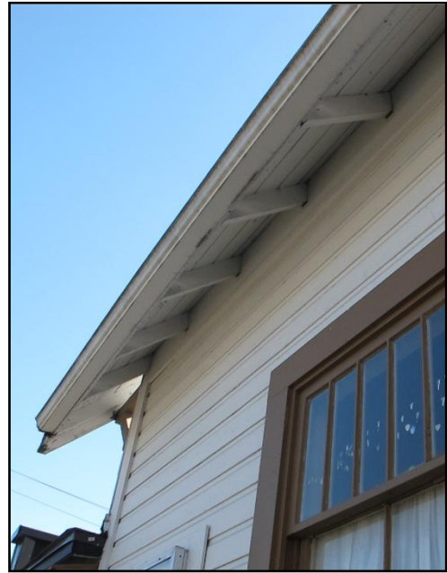
Exposed rafter tails
