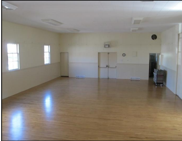
Maple wood floor in main hall
