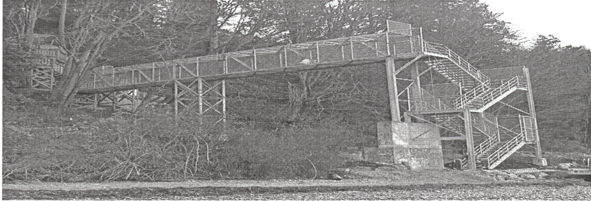
Photo of the Overpass
