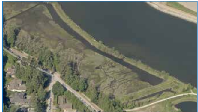
PHOTO: Location of the Stewart Farm Sanitary Pump Station on the south bank of the Nicomekl River
