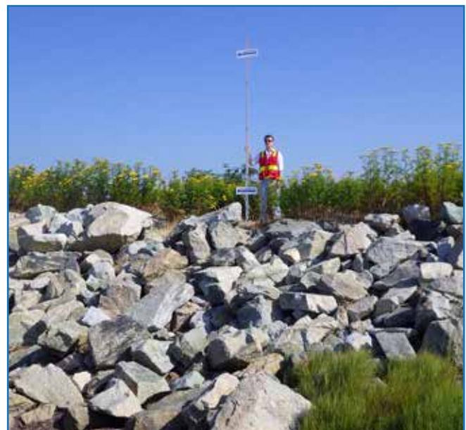
PHOTO: Colebrook Dyke showing Provincial Guidelines for current (lower black line) and future year 2100 elevation (upper black line) targets
