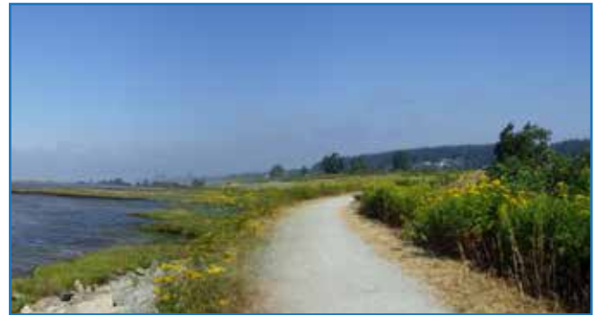
PHOTO: Colebrook Dyke Existing Crest
