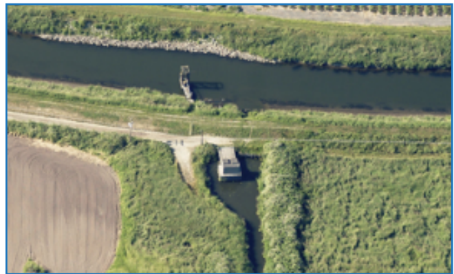
PHOTO: Aerial image of the existing Burrows Drainage Pump Station
