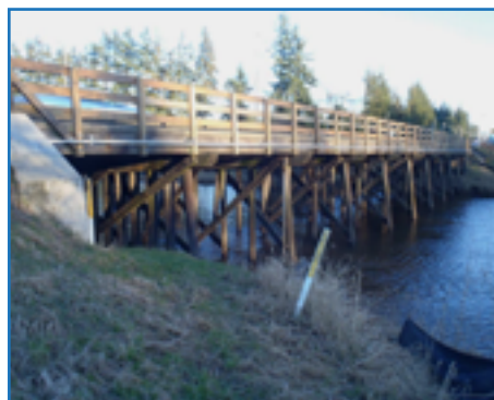
PHOTO: Existing Nicomekl Bridge
