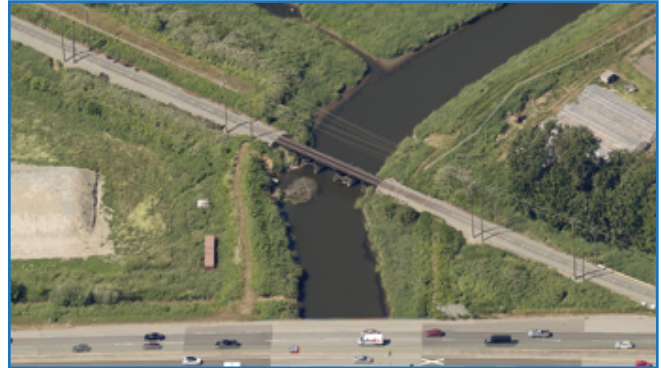
MAP: Aerial image of the existing Serpentine railway bridge
