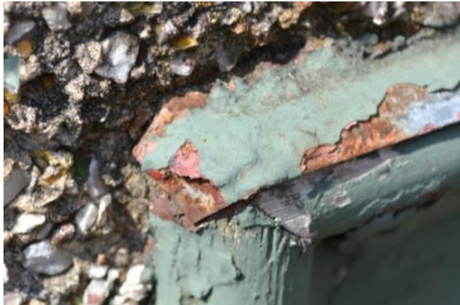
Figure 46: Added metal flashing and wood trim
