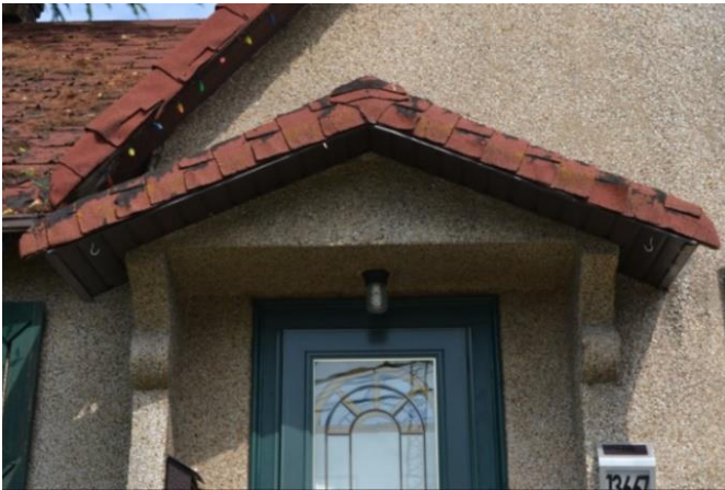
Figure 36: Architectural truss at front gable end
