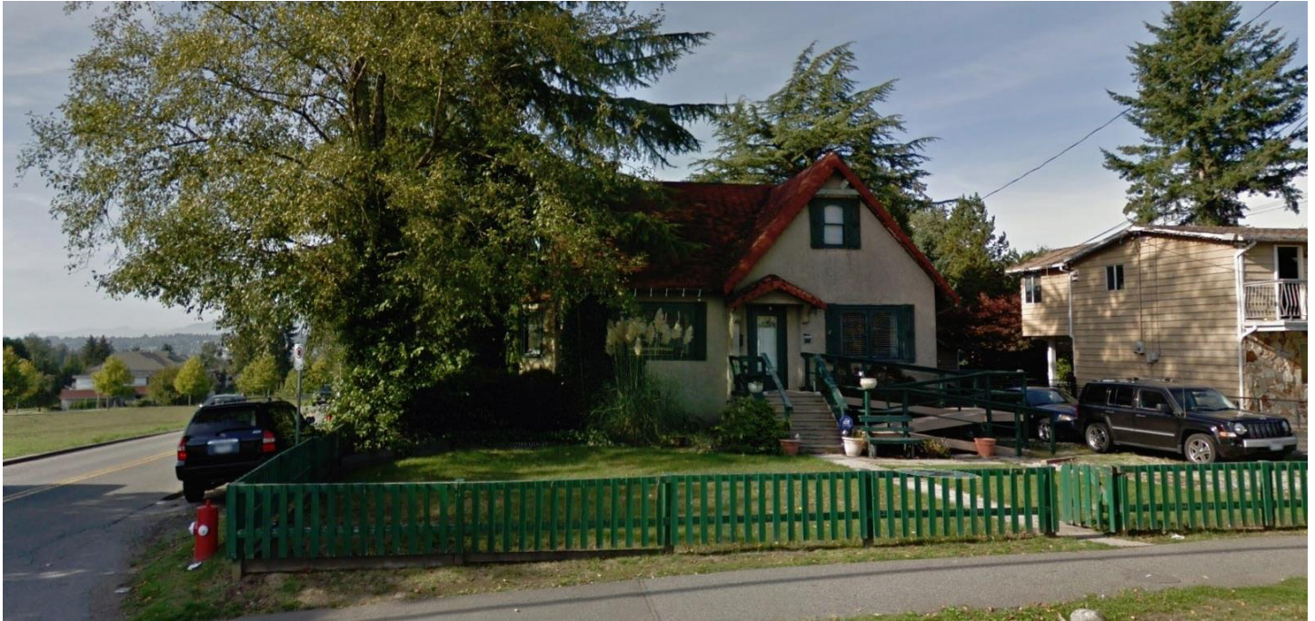
Figure 5: View of the Wixalbrown House from Grosvenor Road at Hilton Road
