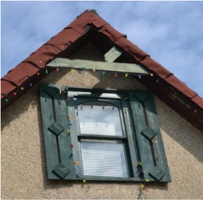
Figure 36: Architectural truss at front gable end
