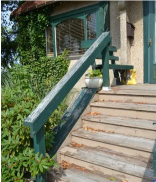
Figure 44: Railing and balustrade
