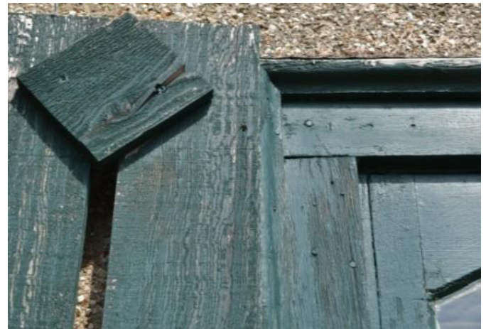
Figure 47: Decorative frame added on top of stucco
