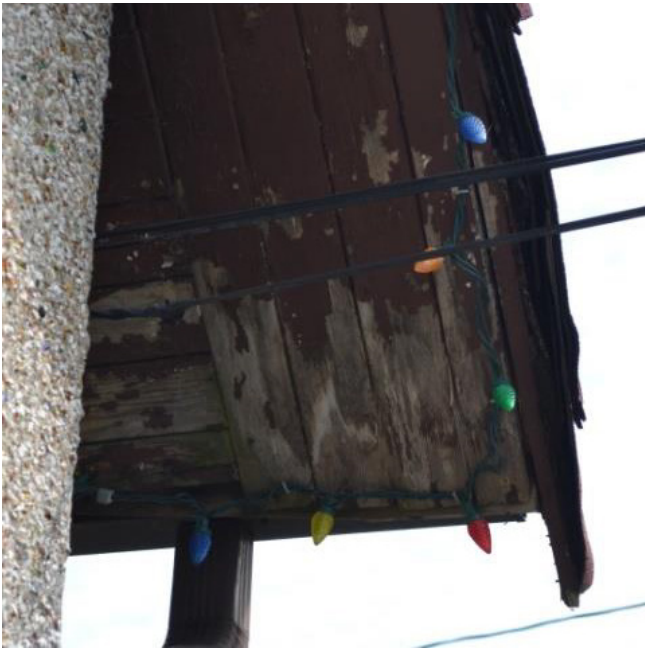
Figure 41: Wood board open soffit
