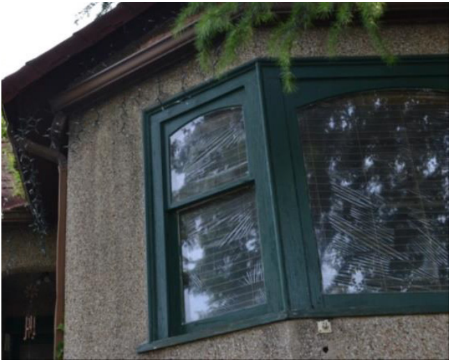
Figure 42: Double-hung window with upper internal arch
