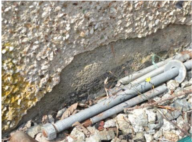
Figure 45: Parging beneath stucco
