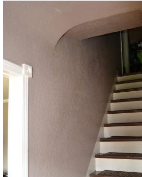
Figure 16: Stairs to second
