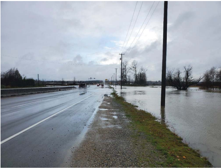
Fraser Highway at 176 St (Northbound)
