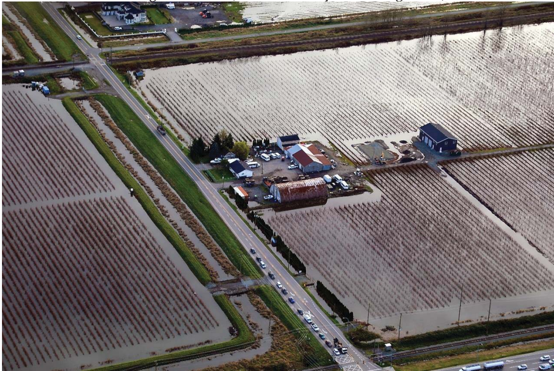
Inter-River area Looking Southwest (168 St and Hwy 10 in Foreground)
