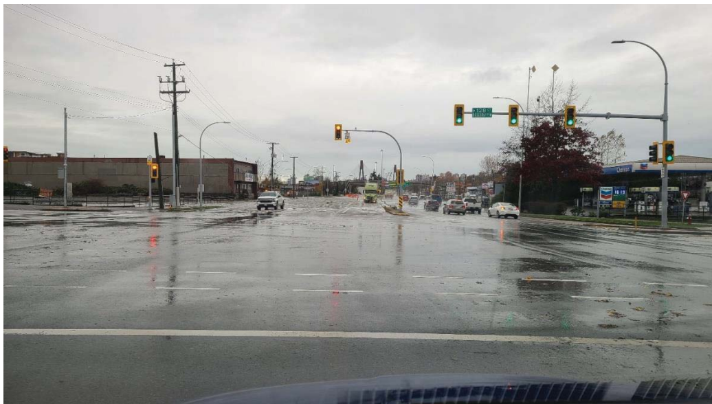
Flooding at King George Blvd and Bridgeview Dr; Looking West on King George Blvd
