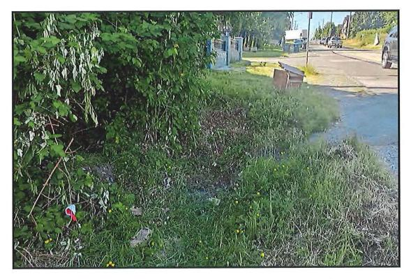
Photograph 4. Roadside ditch that has been abandoned and no longer conveys flow (June 02, 2021).
