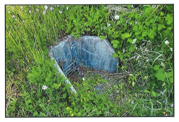
Photograph 5. Inlet to abandoned storm sewer (June 02, 2021).
