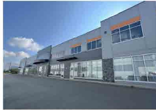
Commercial & Retail development located in 3237 190 St, Surrey
