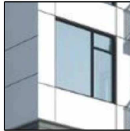
9 Tempered Glass c/w Black Painted Alum Frame
