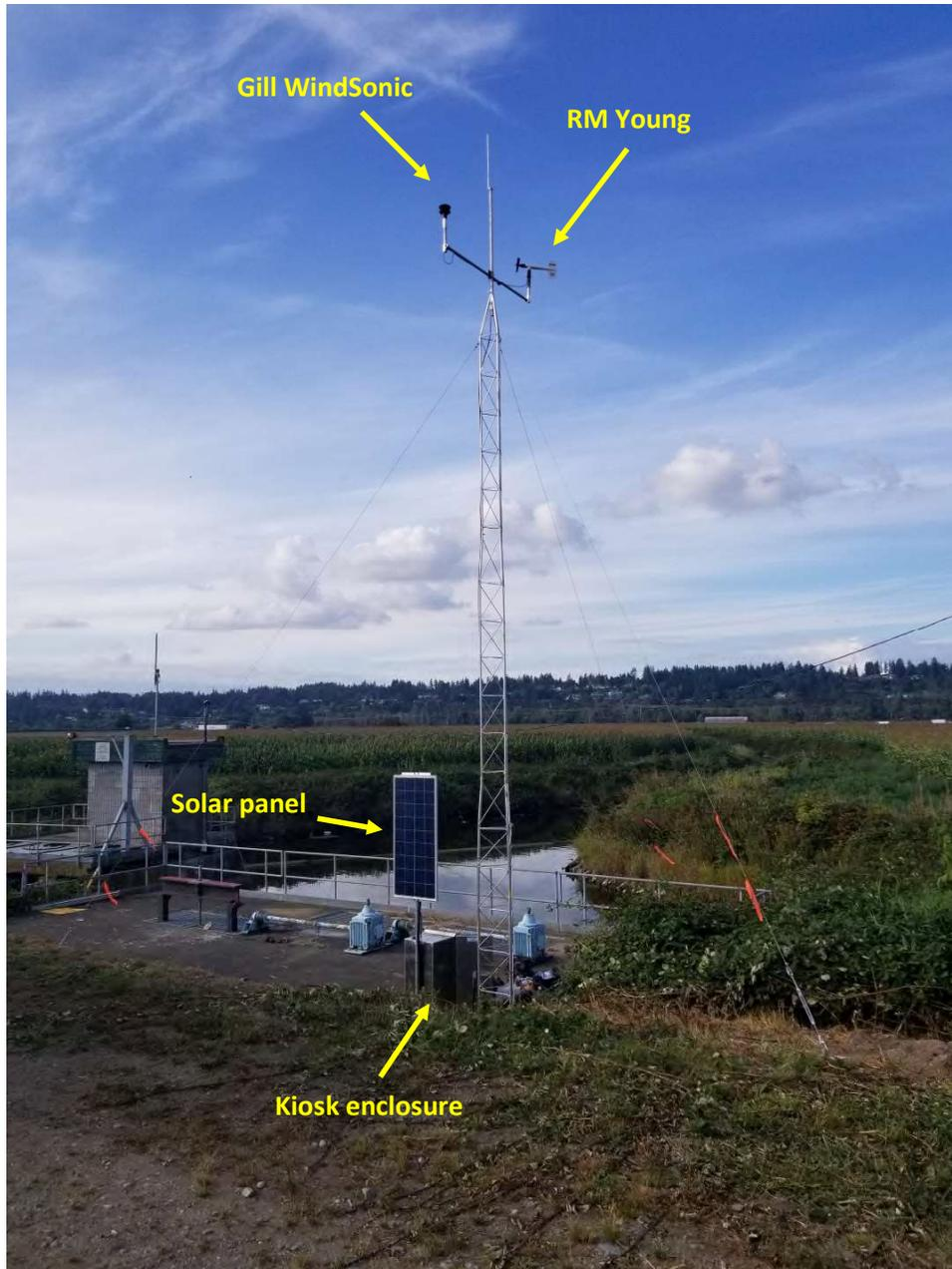
**Photo 2-1 Configuration of the Colebrook Road Pump House Onshore Wind Monitoring Station at the time of installation on 30 August 2019.**
