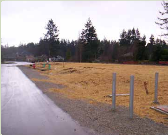
ESC Plans specify the most appropriate BMPs for the site conditions, such as using straw to cover exposed soils to prevent erosion.
