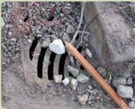
Poorly managed construction sites can result in a considerable amount of sediment entering the City's Drainage system.
