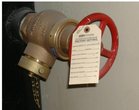
Figure 15 -- PRVs should be marked with the pressure settings and documentation should be kept on site.
