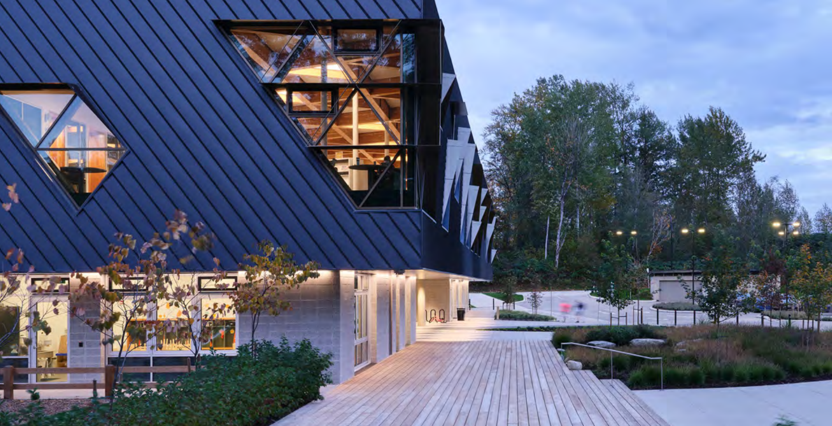
Clayton Community Centre - North America's first Passive House certified community centre (source: @andrewdoraphoto, courtesy of hcma)
