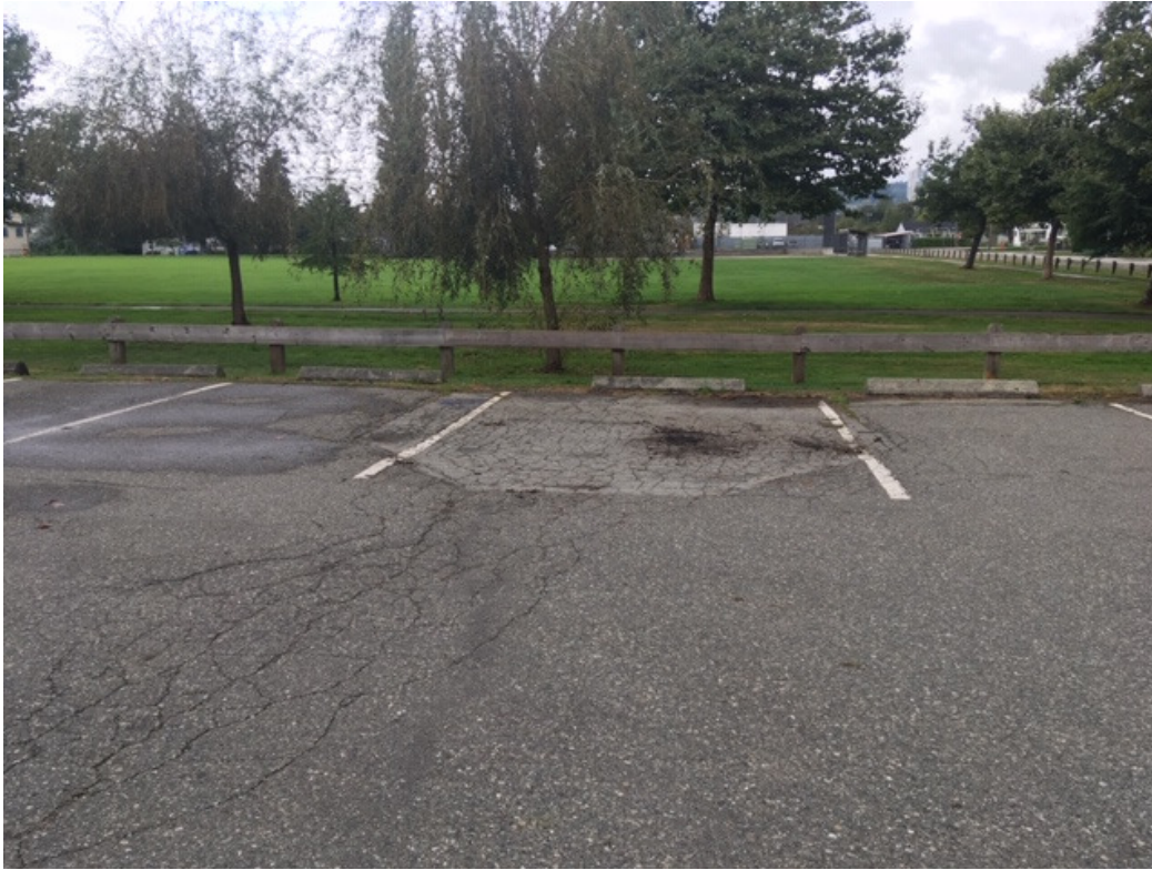
Figure 3: West parking lot, looking west
