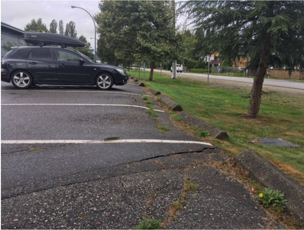
Figure 1: Central Parking Lot looking west.
