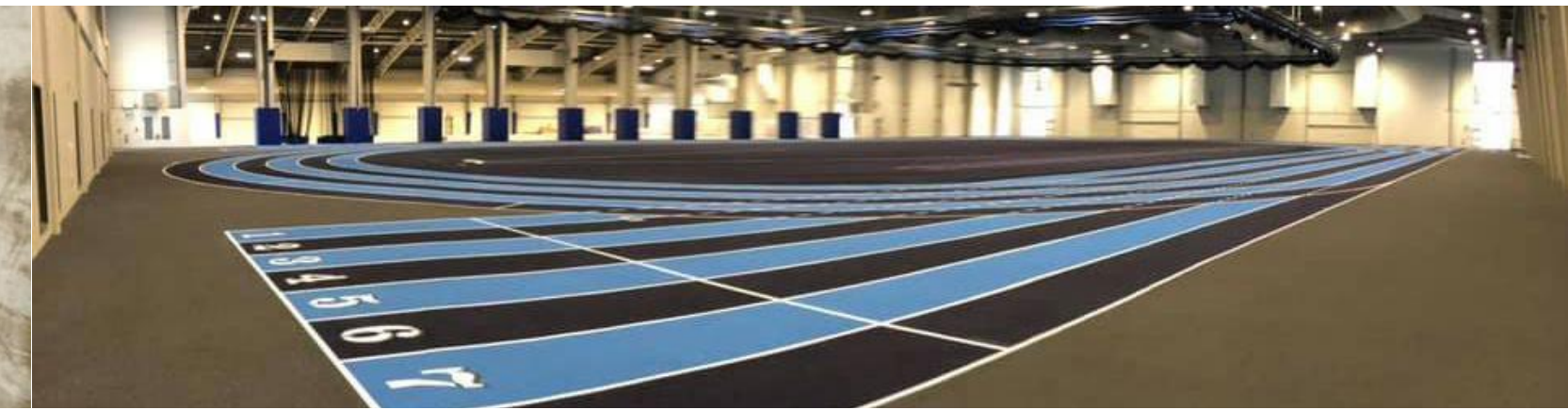
IRVING OIL FIELD HOUSE Saint John, NB BSS 300 • 2019
