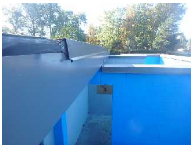
Photo 8: View of exterior fascia. Existing fascia is to be retained, with new metal cap flashings on the roof only. Existing block wall cap flashings are also to be retained.
