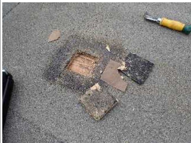
Photo 7: Cut test photo showing 2 ply SBS, 7/16" fibreboard, and kraft laminate vapour retarder.
