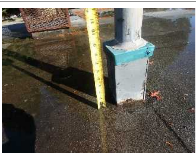
Photo 6: Light post installed in a gum pocket. Anticipate correction and installation of liquid applied membrane solution.
