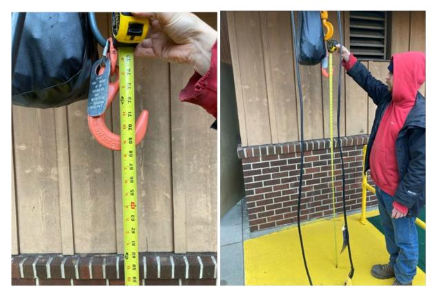
Q9. Can you provide the dimensions of the existing pump specially the existing discharge elbow mounted in the bottom of the wet well? We are looking for the clearance underneath the pump (shown in red below)?
