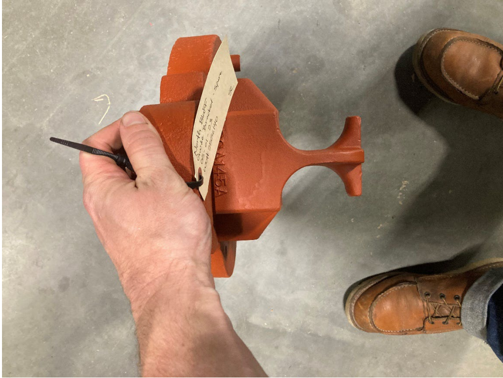
Photo 3: Existing Slide Plate Adaptor
