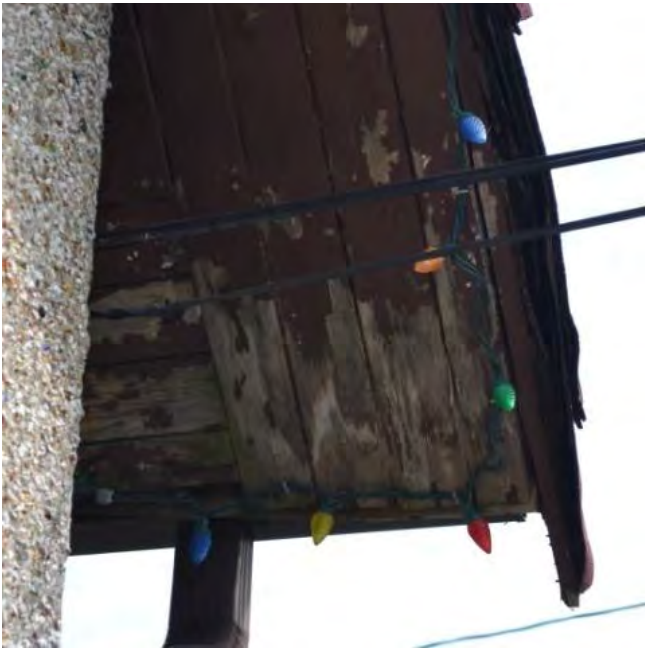
Figure 41: Wood board open soffit
