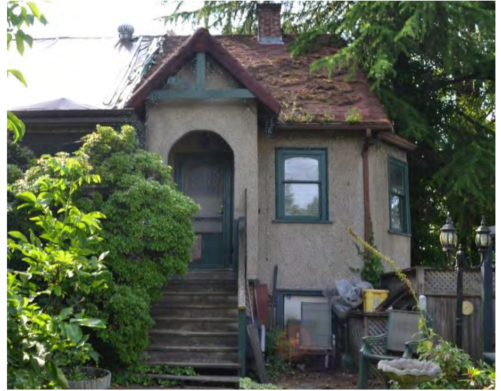
Figure 11: North Elevation; Rear
