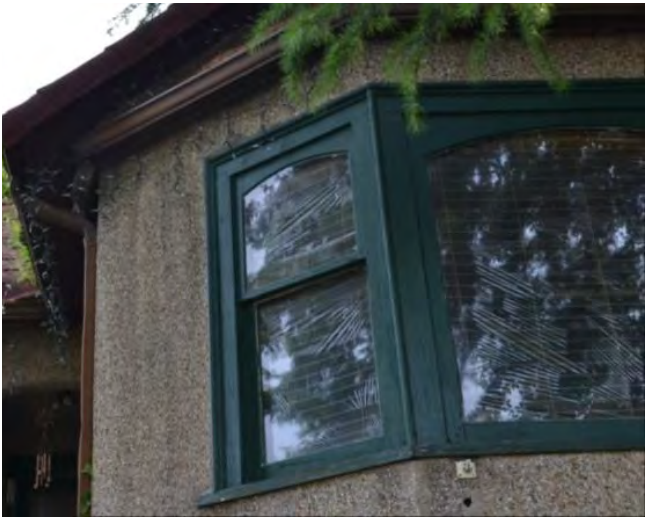
Figure 42: Double-hung window with upper internal arch
