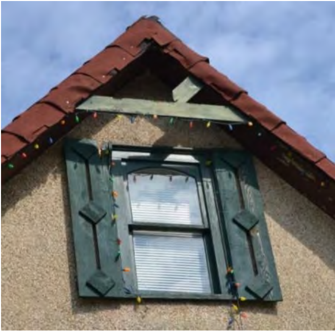
Figure 36: Architectural truss at front gable end
