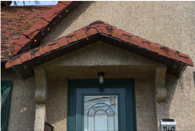
Figure 36: Architectural truss at front gable end
