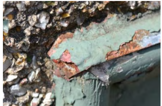
Figure 46: Added metal flashing and wood trim
