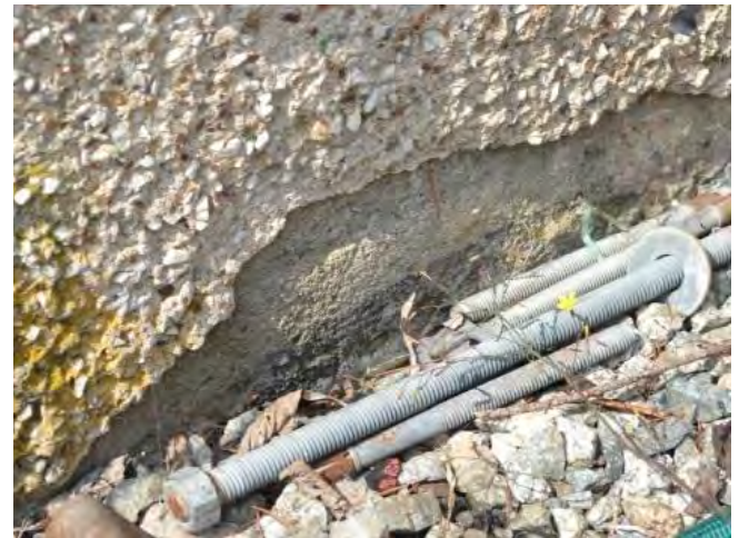
Figure 45: Parging beneath stucco
