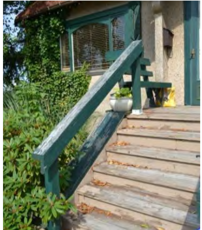
Figure 44: Railing and balustrade
