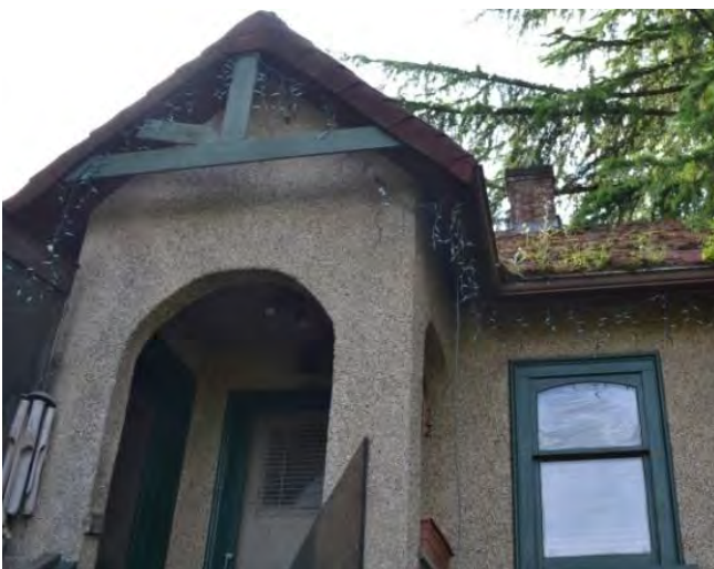
Figure 43: Arched back entrance with architectural truss
