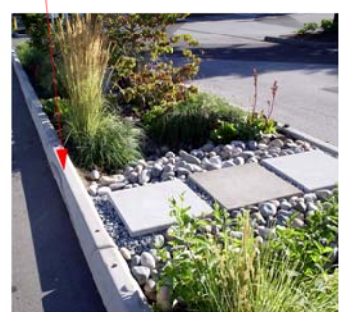
PARKING AREA DRAINAGE STORMWATER MANAGEMENT - VIEW STUDY -TYPICAL CURBED LANDSCAPE STRIP AT PARKING AREA
