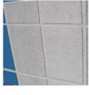
TILT-UP CONCRETE PANEL
