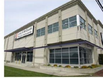
6. VIEW OF ADJACENT SITE ON 104TH AVENUE
