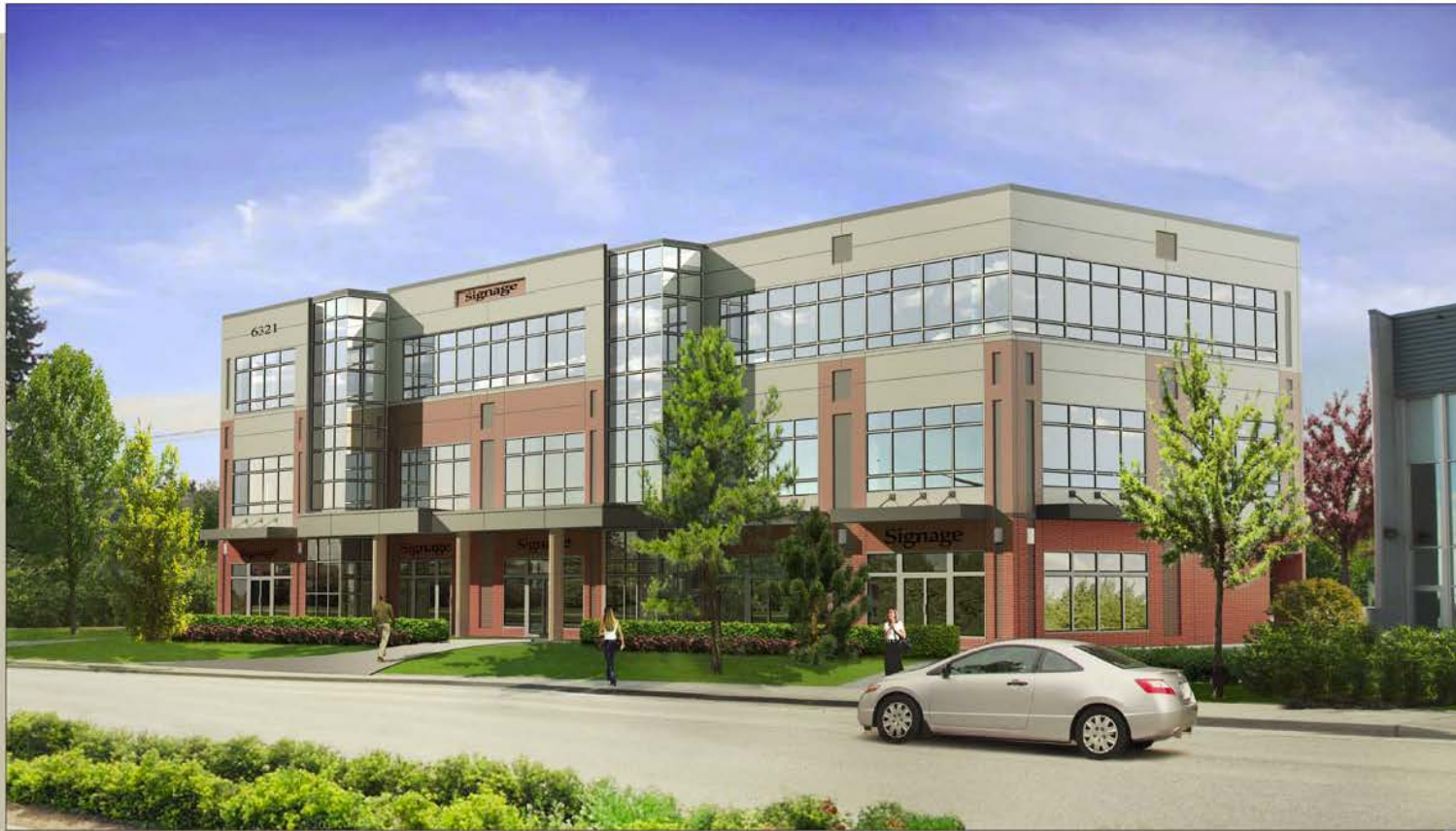
view of building from King George Boulevard
