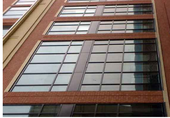
STORE FRONT ALUMINIUM DOOR & WINDOW (MAIN FLOOR)
