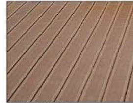
DECK AREA OUTSIDE PAD #8
