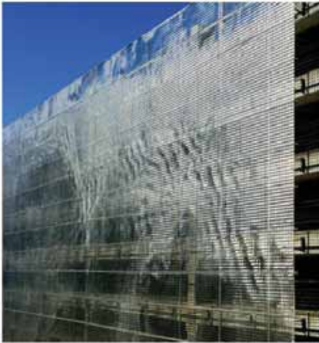
Parking garage, Charlotte, NC
