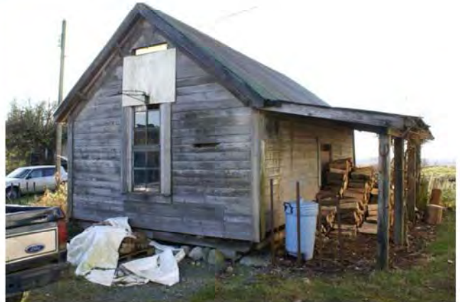
East and north elevations
