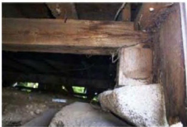
Boulder footing, post and sill beam
