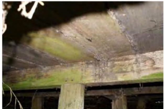
Floor boards resting on structural posts and beams
