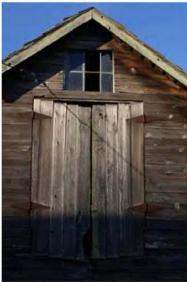
Hinged hayloft doors on south elevation and 6-pane window above
