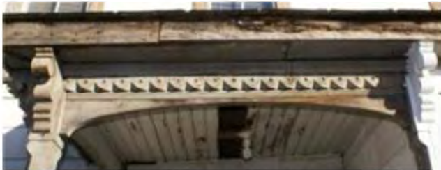
Detail of porch ornamentation: curved beam, dentil pattern carved into beam, and corner brackets.
