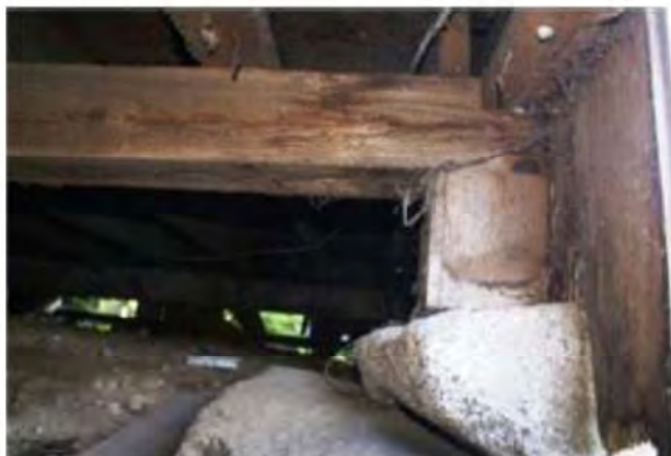
Boulder footing, post and sill beam
