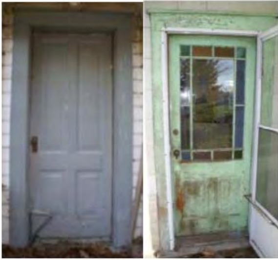
Existing wood doors
