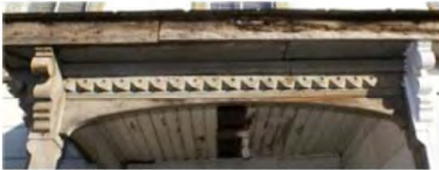
Detail of porch ornamentation: curved beam, dentil pattern carved into beam, and corner brackets.
