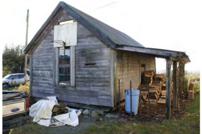
East and north elevations
