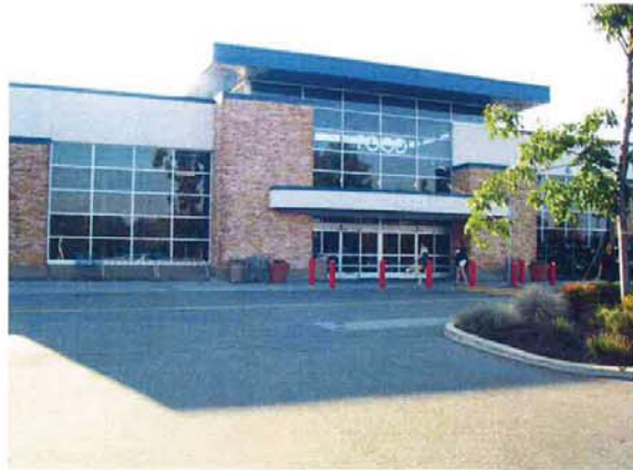
BEFORE - NORTH ELEVATION EAST
