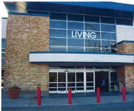
BEFORE - EAST ELEVATION
