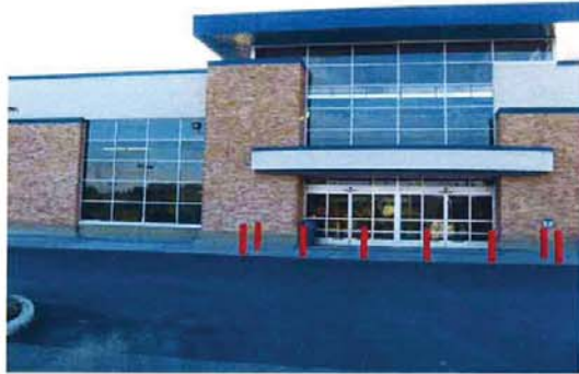
BEFORE - EAST ELEVATION
