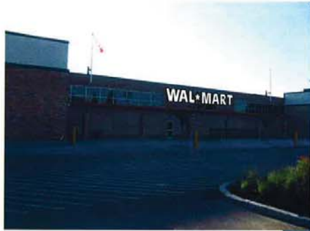
BEFORE - EAST ELEVATION
