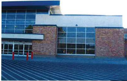
BEFORE - EAST ELEVATION
