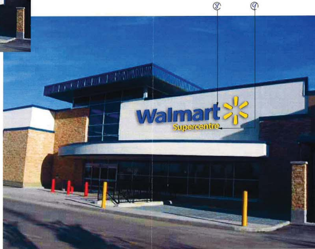
AFTER EAST ELEVATION NORTH
