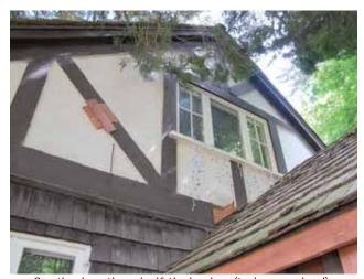
South elevation: half-timbering (to be repaired), wood trim and projected sill
