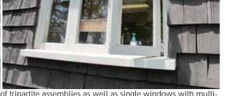
Additional original window assemblies – note the presence of tripartite assemblies as well as single windows with multipaned transoms
