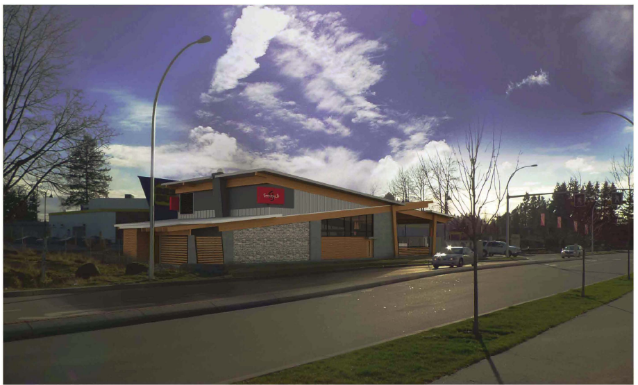
2 VIEW FROM CROYDON DRIVE HEADING WEST
