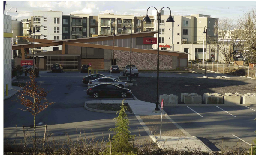
2 VIEW FROM 24TH STREET
