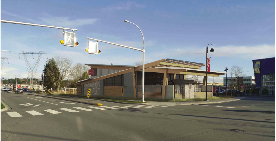
1 VIEW FROM CROYDON DRIVE HEADING EAST
