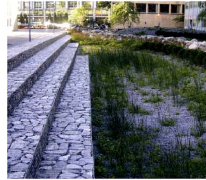
Precedent: Dry rock detention channel with planting
