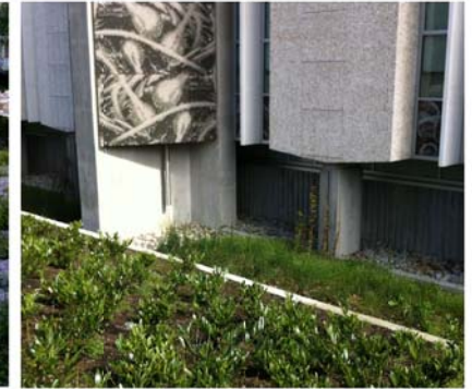
Precedent: Exposed rainwater leader
