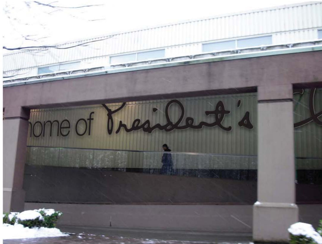
B NEW NON-ILLUMINATED REVERSE CHANNEL LETTERS X1 NOT TO SCALE
