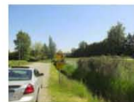
Streetscape View Existing ditch adjacent to Highway 99
