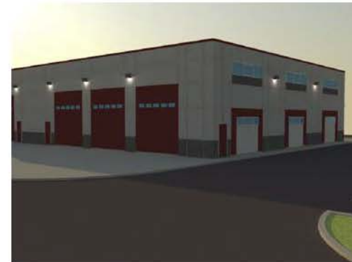
VIEW OF PHASE 1 BUILDING FROM SOUTHEAST
