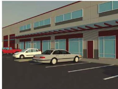
VIEW OF PHASE 2 BUILDING FROM NORTHWEST
