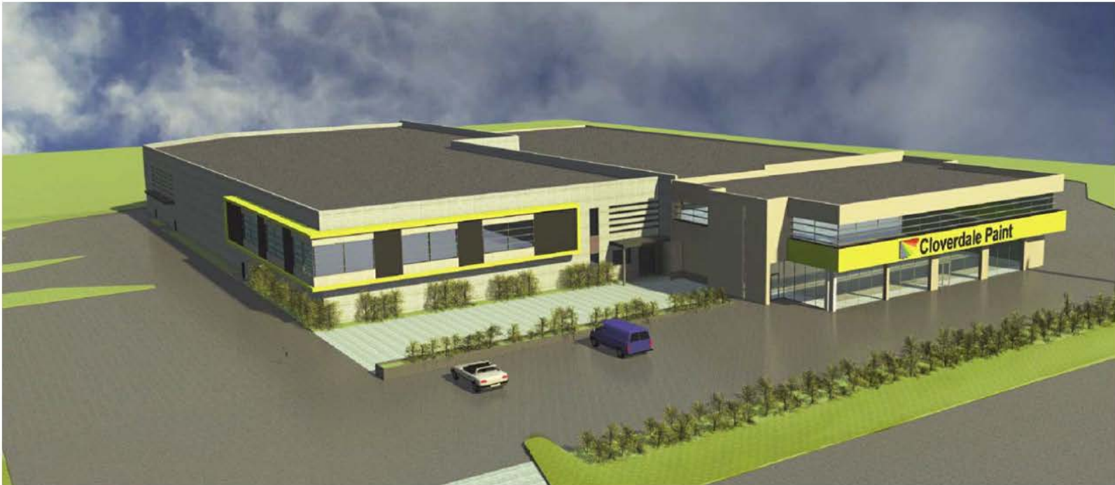
BIRD'S EYE VIEW OF ENTIRE BUILDING
