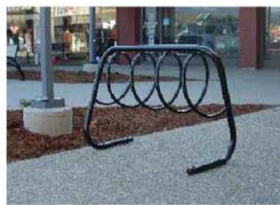
4. BICYCLE RACK ON CONCRETE PAD (1200 X 1800 X 75) WITH 100 X 100 X 75 CONCRETE PAVERS
