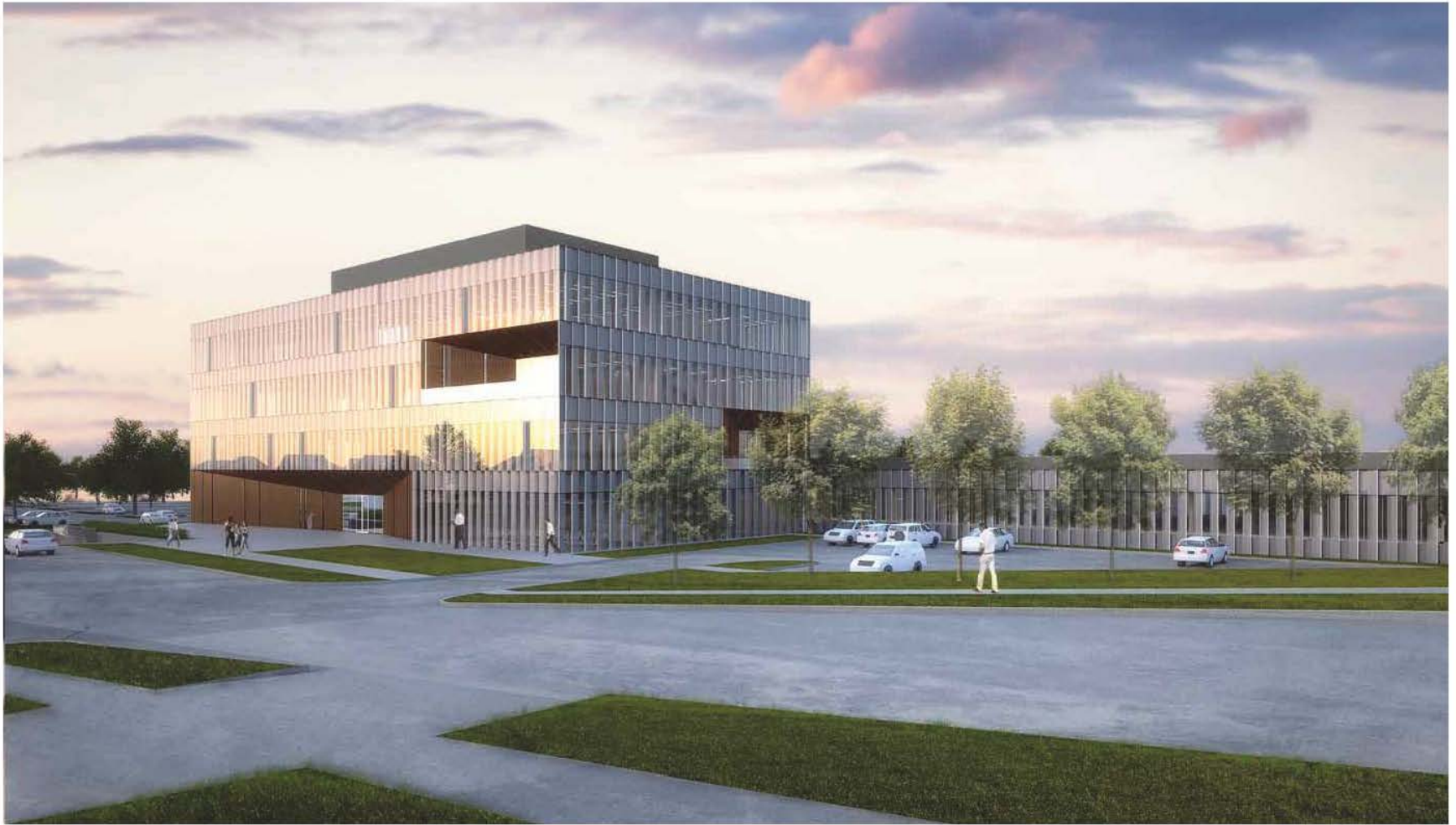
NORTH EAST OPERATIONS CENTRE FROM 148TH STREET
