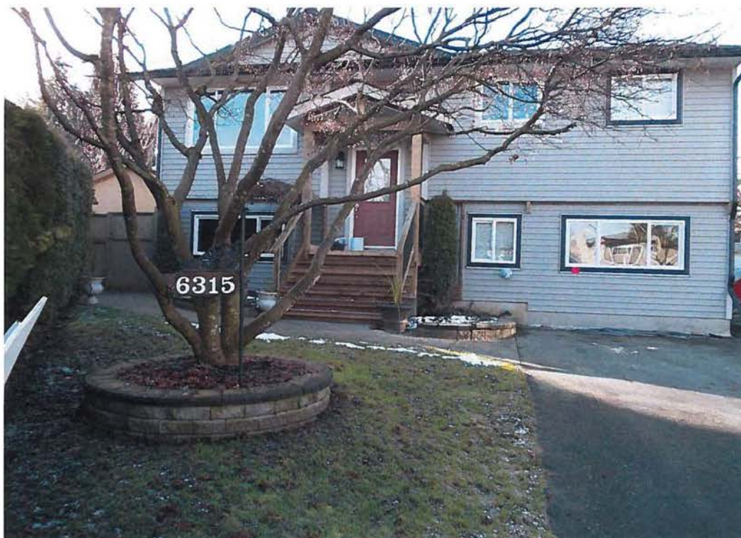
House after filling in the garage.
