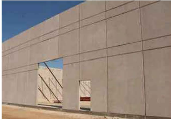
TILT-UP CONCRETE WALL PANEL
