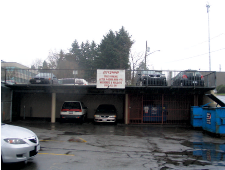
EXISTING DISPLAY- TYPICAL
