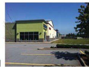
SOUTHEAST CORNER OF ADJACENT BUILDING TO THE WEST
