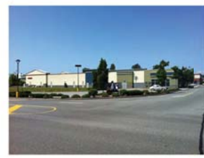
SITE AND ADJACENT BUILDING TO THE WEST
