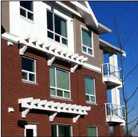
View of Existing Bldg. K with Shading Devices, Hardie Panel, Metal & Glass Railings, Brick and Hardie Clad Columns
