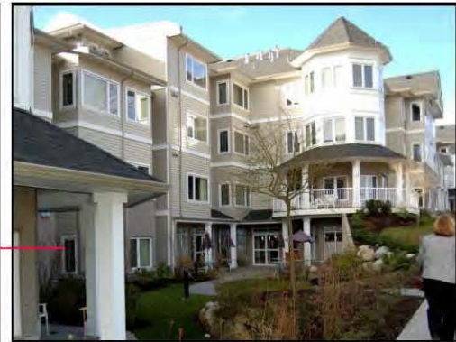
View of Building E
