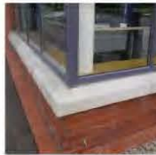
Precast Concrete sills/Masonry Caps
