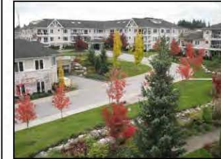
View of Bldg. C, D & Amenity Bldg.
