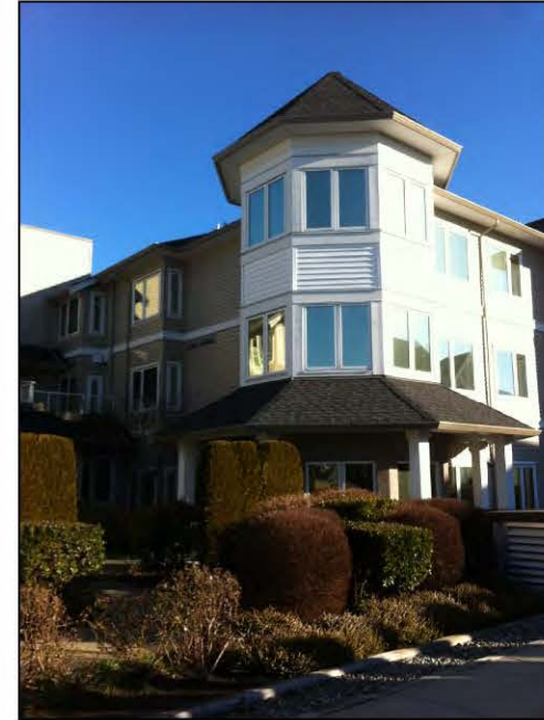
View of Existing Bldg. E
