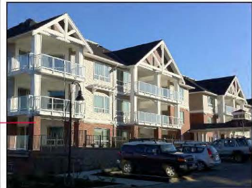
View of Building K
