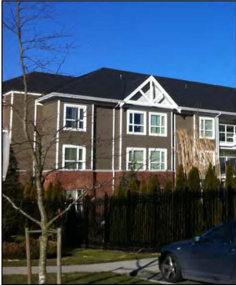
View of Existing Bldg. H & Metal Gate Enclosed Gardens
