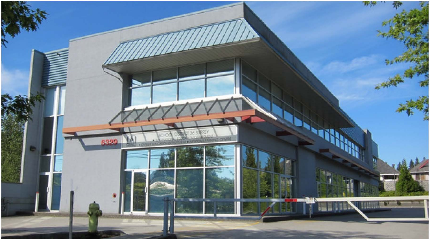
SITE PHOTO: 6329 King George Blvd
