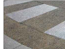
CONCRETE WITH DECORATIVE COLOUR BANDS
