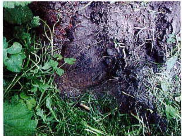
Photo No.08: Soil conditions at bottom of slope Approximately 0.3m of topsoil and vegetation over glacial till
