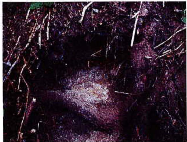
Photo No.04: Soil conditions at top of slope Up to 0.3m of topsoil and vegetation overlying glacial till
