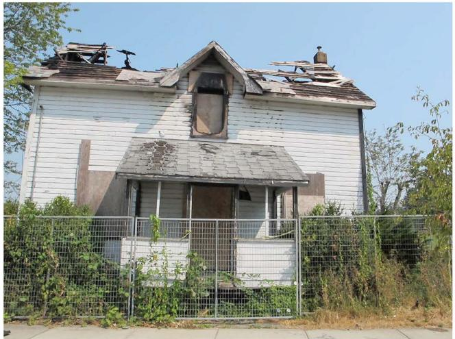
Photo 8: West Elevation, fire damage in 2010.
