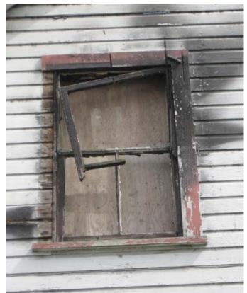
Photo 13: Typical 2-over-2 double-hung wood sash window with trim and sill, 2012.
