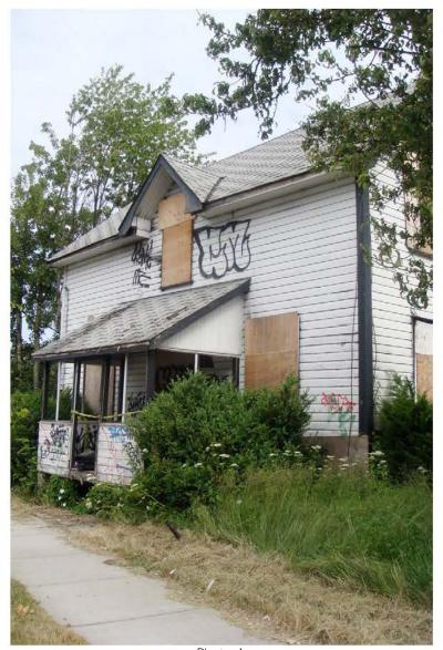
Photo 4: Front Elevation (south) showing cross gable dormer; entrance porch with shed roof; whalebone bargeboards; closed soffits and corner boards, 2009.
