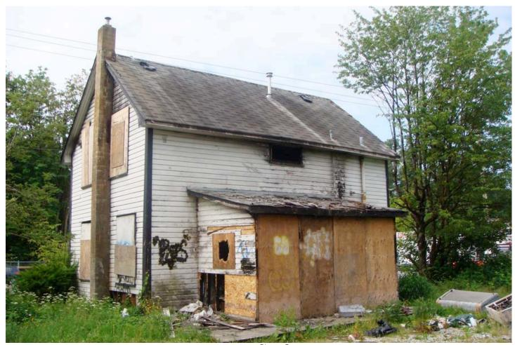
Photo 5: Rear Elevation (north) showing extensive fire damage; and enclosed shed roof addition, 2009.
