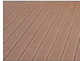
DECK AREA OUTSIDE PAD #3
