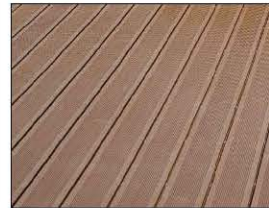
6 L4 DECK AREA OUTSIDE PAD #3
