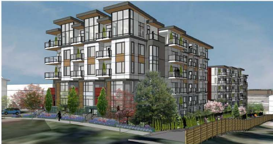
BUILDING 2 - NORTHEAST CORNER
