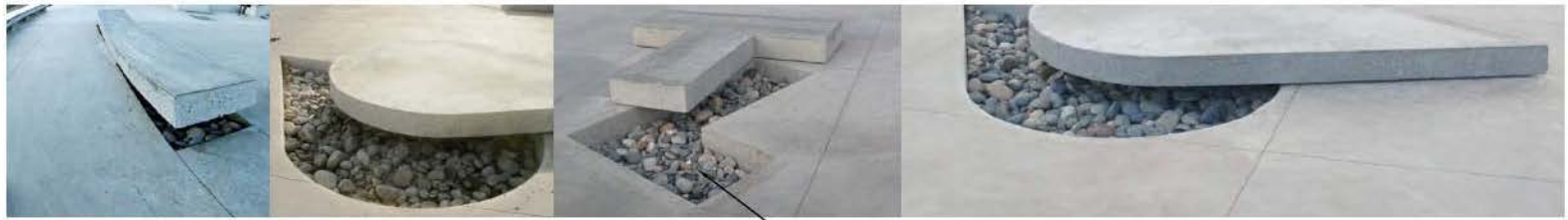
PRECEDENT IMAGES OF CONCRETE OFFSET TO REVEAL GRAVEL BASE. REVEAL CAN ALSO BE PLANTED WITH SHRUBS OR GRASSES.
