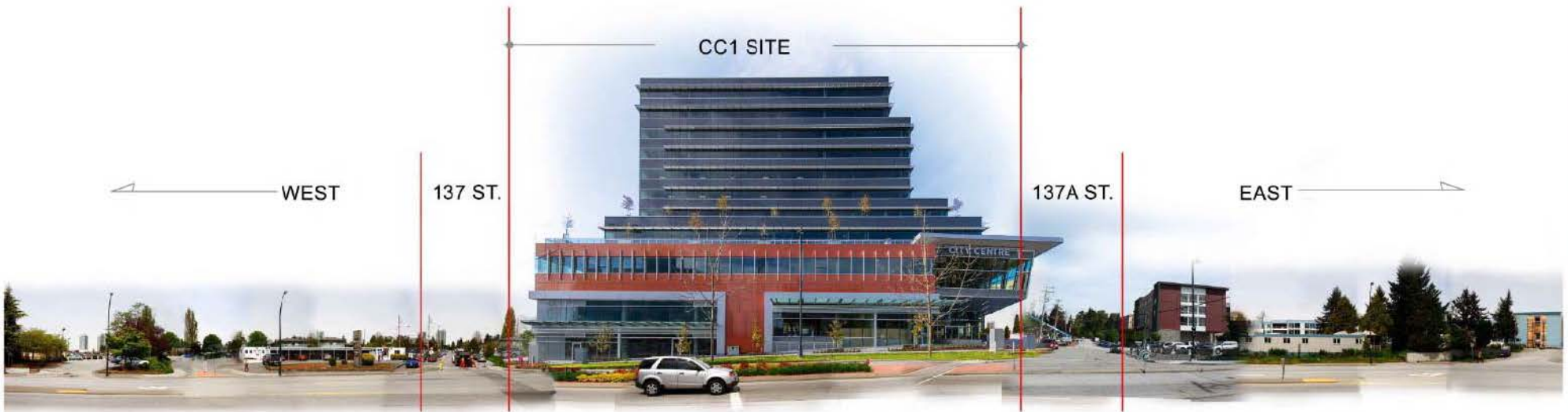
VIEW FROM 96TH AVE. LOOKING NORTH
