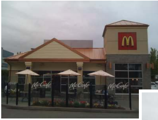
BEFORE - EAST ELEVATION
